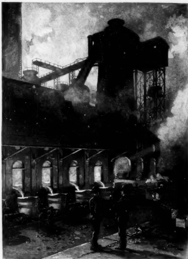
A MODERN BLAST-FURNACE, BESSEMER, PENNSYLVANIA—TAPPING THE FURNACE INTO LADLES.
